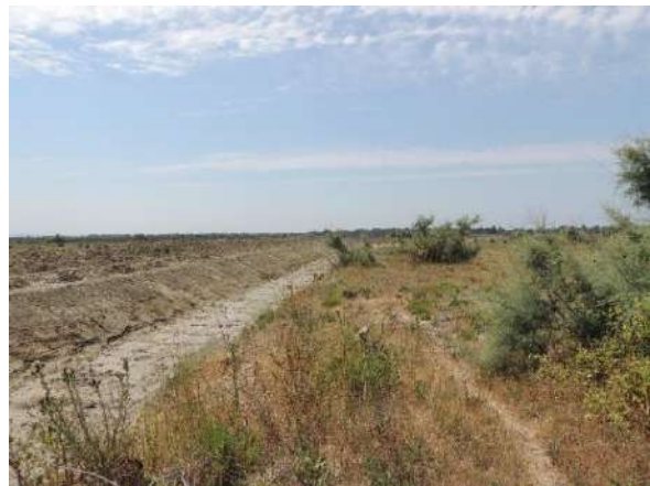
Figure 80. Drainage channel inside the PDA area, recently maintained with removal of vegetation along the bank (WP007, heading South) (Fauna Datasheet- Picture 8517).
