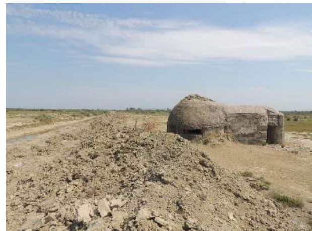
Figure 84. Bunker along the drainage channel (WP009. Heading North): bats activity (droppings) was observed inside the bunker during summer visit in PDA (August 2020) (Fauna Datasheet- Picture 8526).
