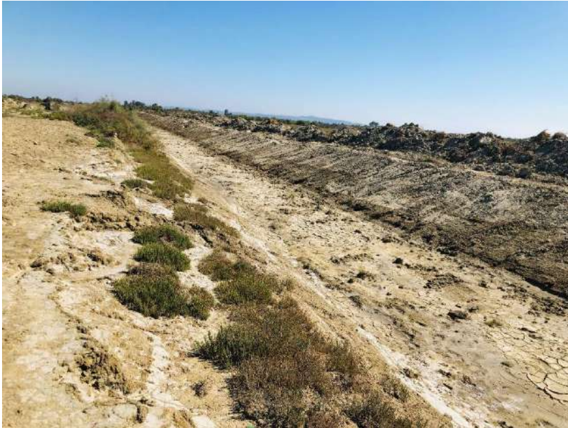
Figure 28. Irrigation Channel in the PV Area
