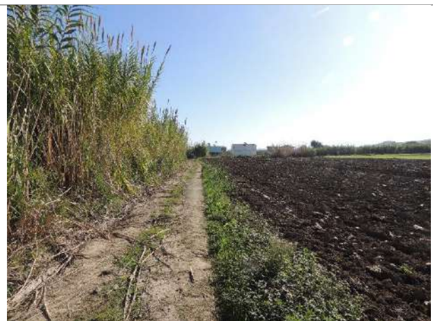
Picture 623. TL220 kV heading towards Fieri Sub Station, passing through arable lands, with hedges of Arundo donax (WP032, heading E)
