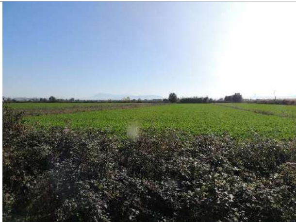
Picture 593. TL 220 kV Fier-Hoxhare alignment passing through arable land (WP028, heading South)
