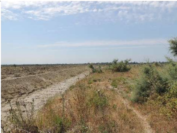
Picture 8517. Drainage channel inside the PDA area, recently maintained with removal of vegetation along the bank. (WP007, heading South)
