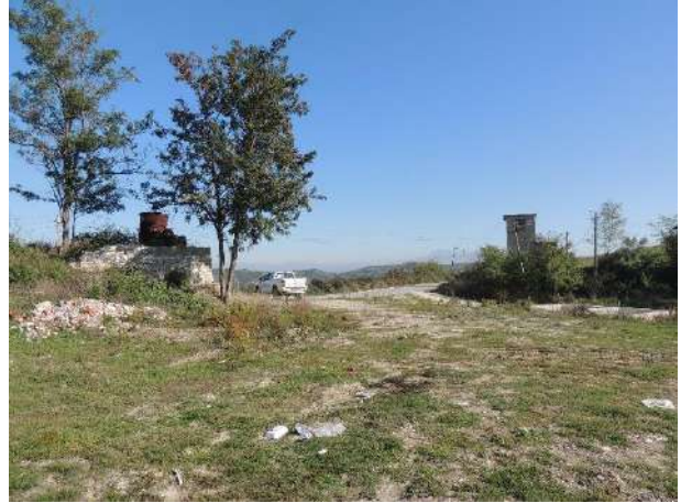
Picture 681. TL220 kV heading towards Fieri Sub Station, intersection with access road to Peshtan (WP038, heading SE)
