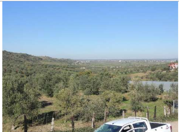
Picture 661. TL220 kV heading towards Fieri Sub Station, passing through gentle hills covered with olive groves (WP036, heading North)
