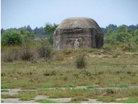
Figure 103. Bunker serving as a possible nesting site for the Little Owl
