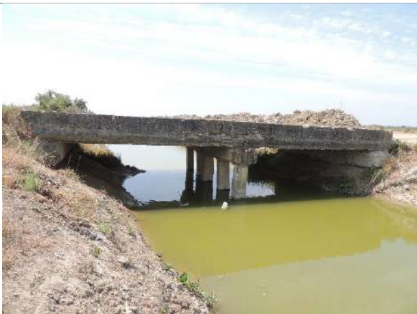
Picture 8537. Bridge over a drainage channel inside the PDA. WP010 (heading NE)
