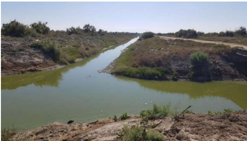
Figure 26. Views of the second range drainage channels in the project area
