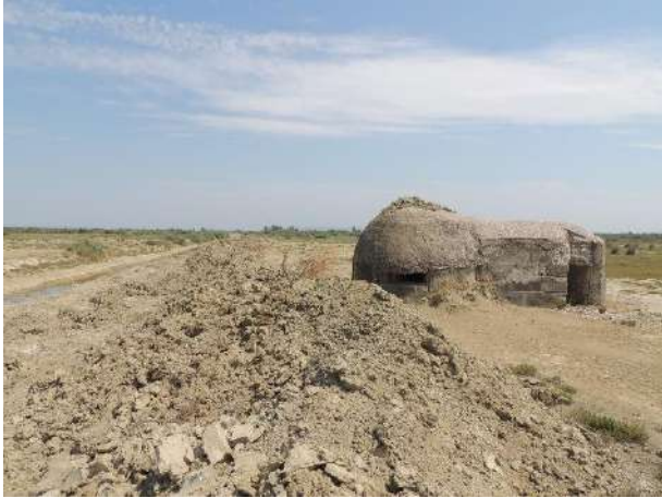
Picture 8526. Bunker along the drainage channel (WP009. Heading North)
