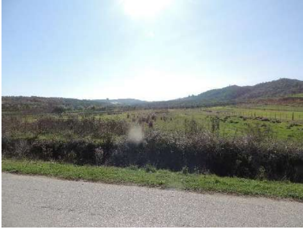
Picture 648. TL220 kV heading towards Fieri Sub Station, passing through arable lands and gentle hills covered with olive groves (WP034, heading South)
