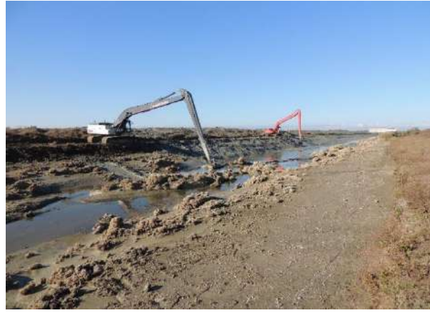
Figure 82. Cleaning operations under way along the secondary drainage channel, parallel to Emisari i Myzeqese (WP005, heading West), (Fauna Datasheet- Picture 386).
